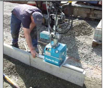
Turbo M-Levator with suction plate GG 80 – edging stone
